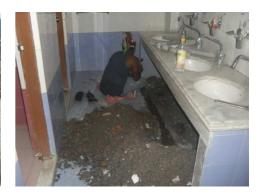
The beginning of the year saw a lot of work in our Home. Merely a year after moving into the Building, walls of the stairwell were so saturated that water dripped down the bathroom walls. The cause, though, could not be found, and we took the drastic measure of replacing all water and drainage pipes. This took over two weeks to do and cost appr. 950 SFR. We now hope to have solved the leakage problems.
